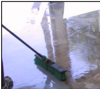
Use a Broom to Scrub Surface
